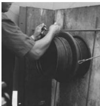
5. For additional stability, it's necessary to secure the sleeve with wire to the rebar. Insert the other end cap firmly, check that second end cap is positioned correctly, confirm sleeve length and close the form.
