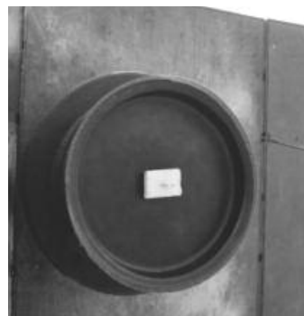
Place second cap on the sleeve and use a (block of wood*) and (wing nut*) to tighten unit in place. Make certain sleeve is plumb.
